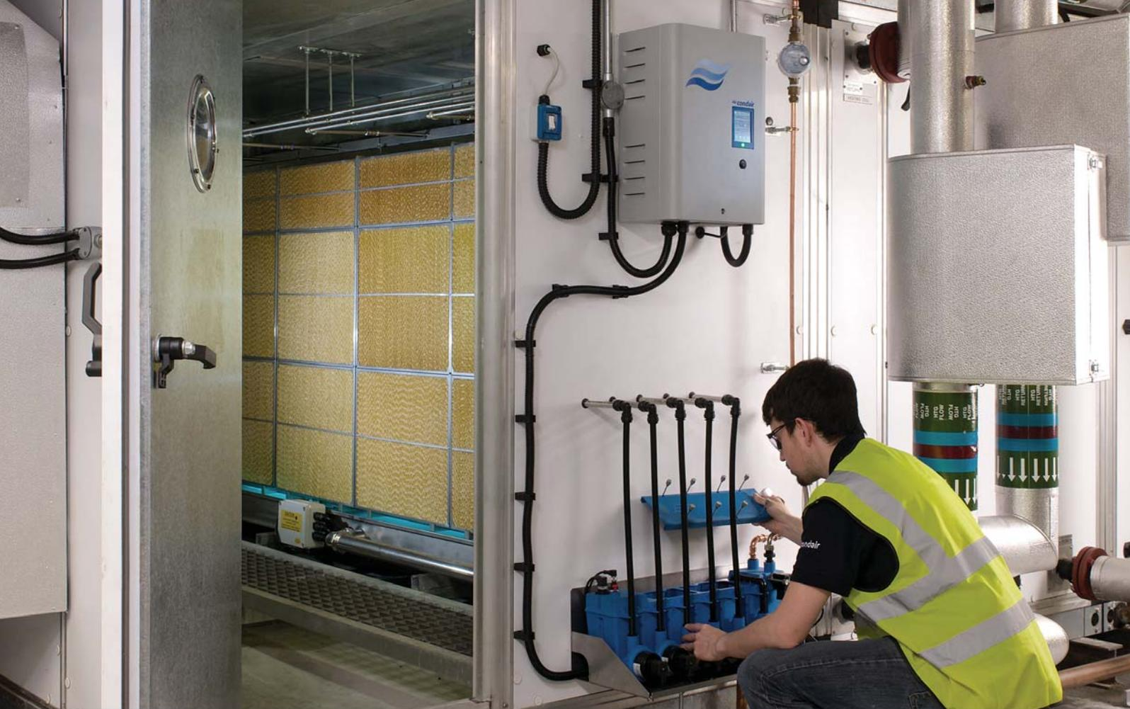
Condair ME with externally mounted hydraulic unit
