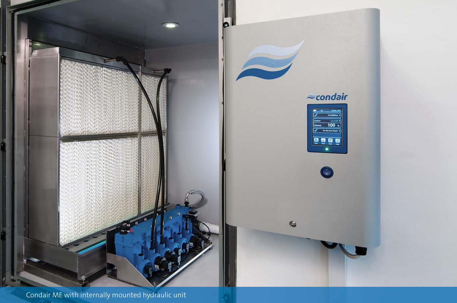
Condair ME with internally mounted hydraulic unit
