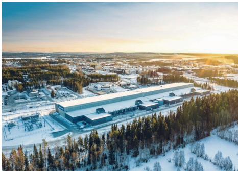
Facebook Datacentre, Lulea, Sweden
